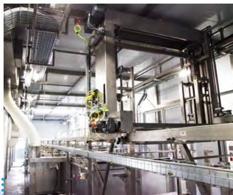
Trolley detail Dip washing line for axle components
