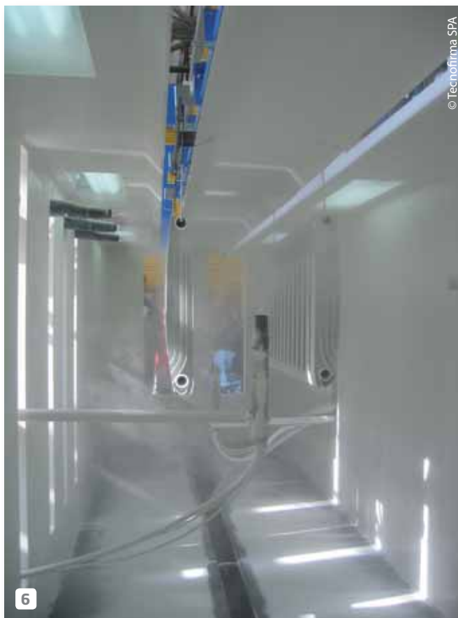
6 The powder application process. The hanger remains outside the booth to ensure it is always clean.
